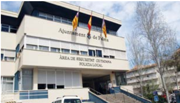
Directorate General Building of Police of Palma de Mallorca (Spain)
