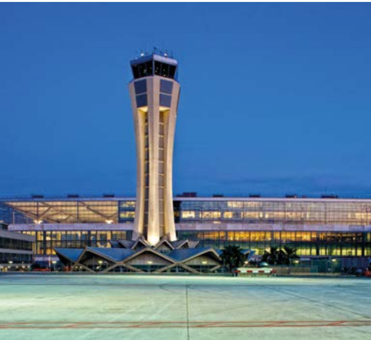
Replacement and updating of air-conditioning and fire protection systems at Malaga – Costa del Sol Airport (Spain)
