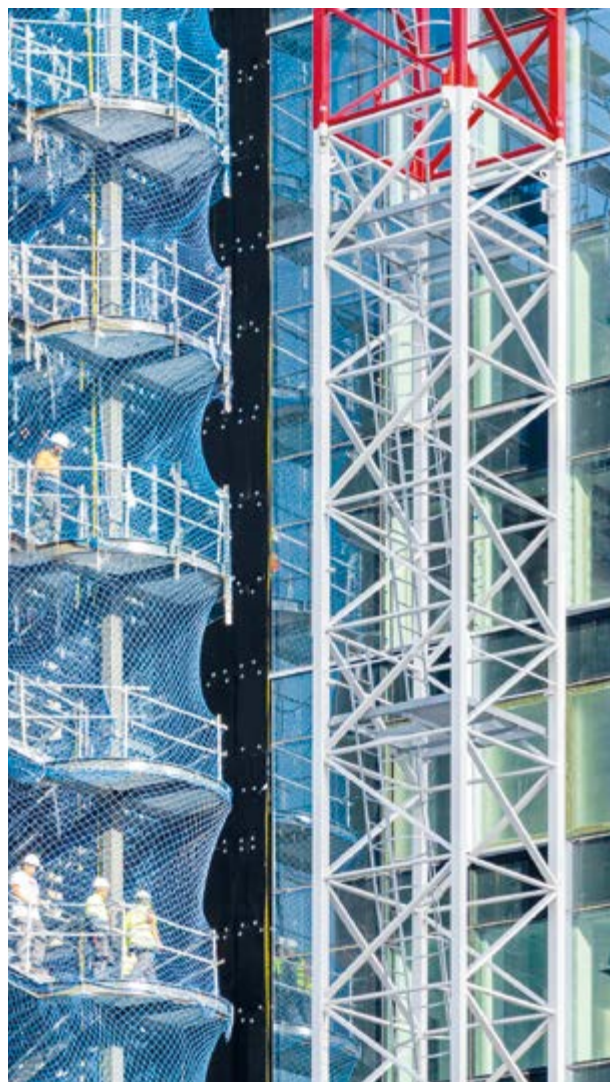
Office Building of Generali at 4, Orense St., AZCA - Madrid (Spain)
