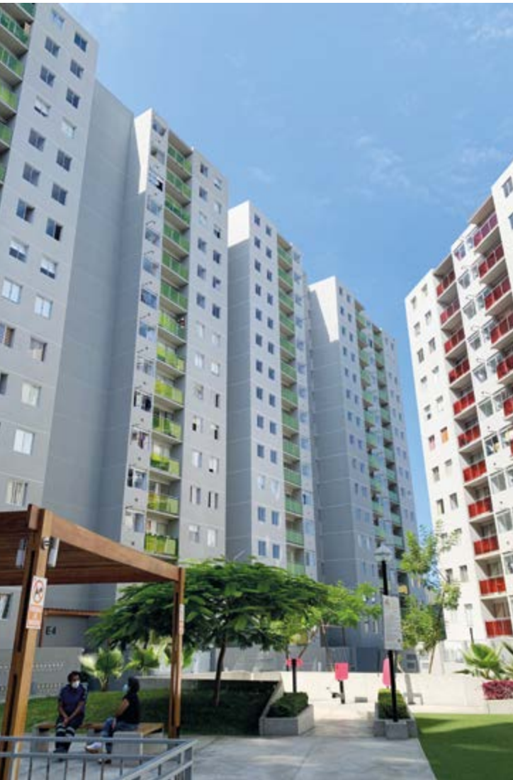
Nuevavista Condominium in the district of Bellavista in the Province of Callao 1,104 housing units-, Lima (Peru)
