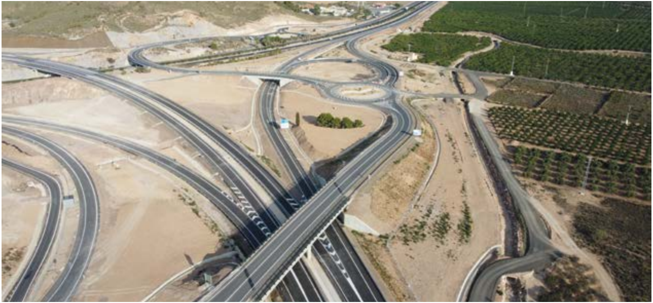
Stretch Junction of La Concepción – Junction of the A7 Mediterranean Dual Carriageway, Almería (Spain)
