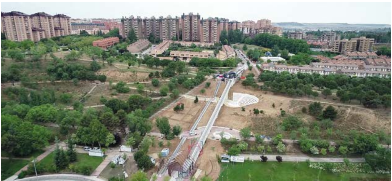
Vertical mobility and mechanical lifts on the Eastern slope of the Parquesol neighbourhood, Valladolid (Spain)
