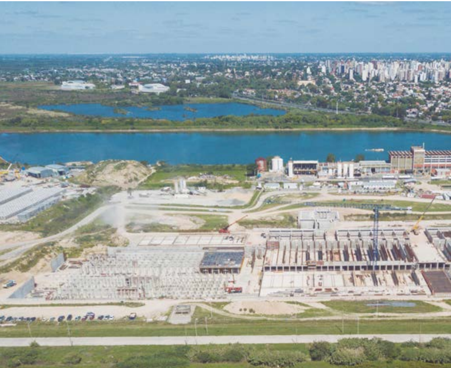
Station d'épuration de General Belgrano, Buenos Aires (Argentine)
