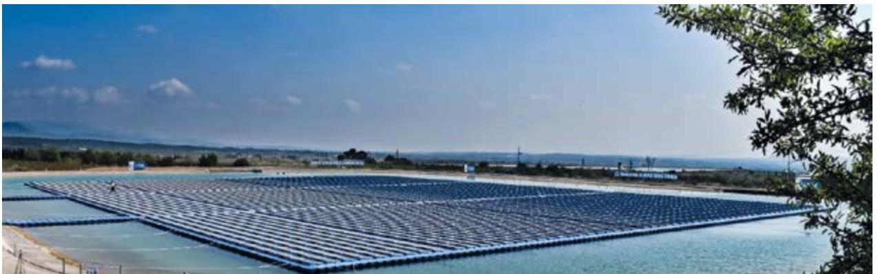
Floating solar pumping on raft and two underground pumps for the self-consumption of the Irrigation Community of Liria, Valencia (Spain)
